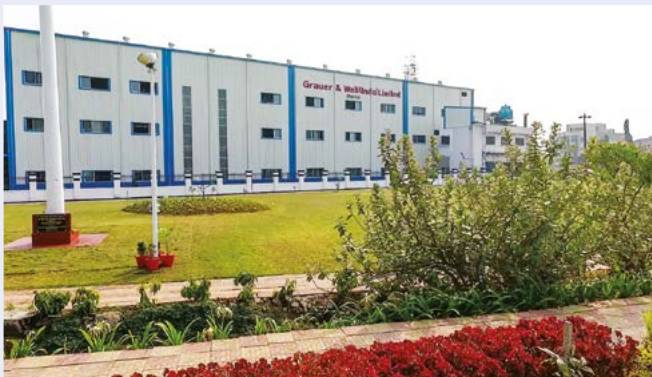
Dadra Paints Plant Western India
