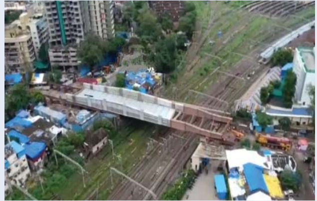
Launch of Hancock railway overbridge between Sandhurst Road and Byculla stations on main line of Central Railway
