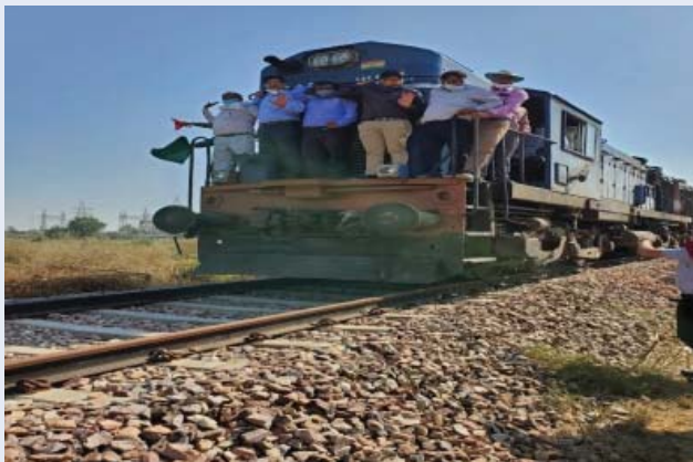
Commissioning of railway siding of CONCOR at MMLP Barhi, Sonapat
