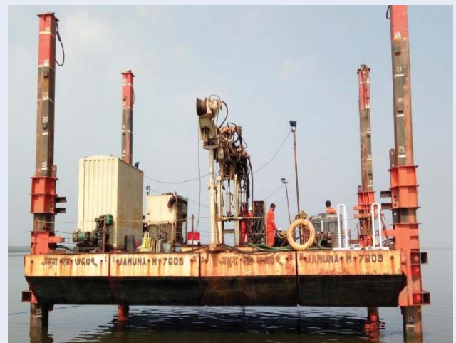
Drilling for undersea tunnel through jack-up rig at Thane creek for Mumbai- Ahmedabad HSR Project
