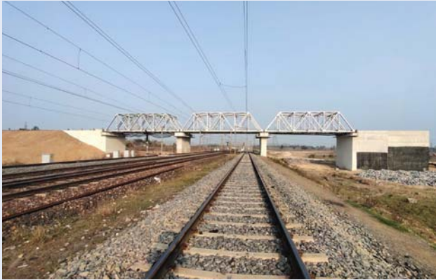
Rail Over Rail Bridge on Howrah-Mumbai Main Line for OPGC MGR project
