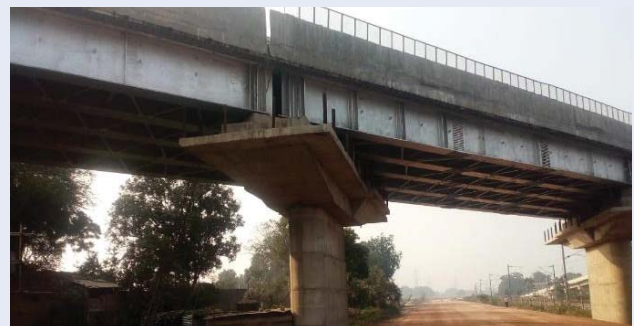
Road Over Bridge for DFCCIL
