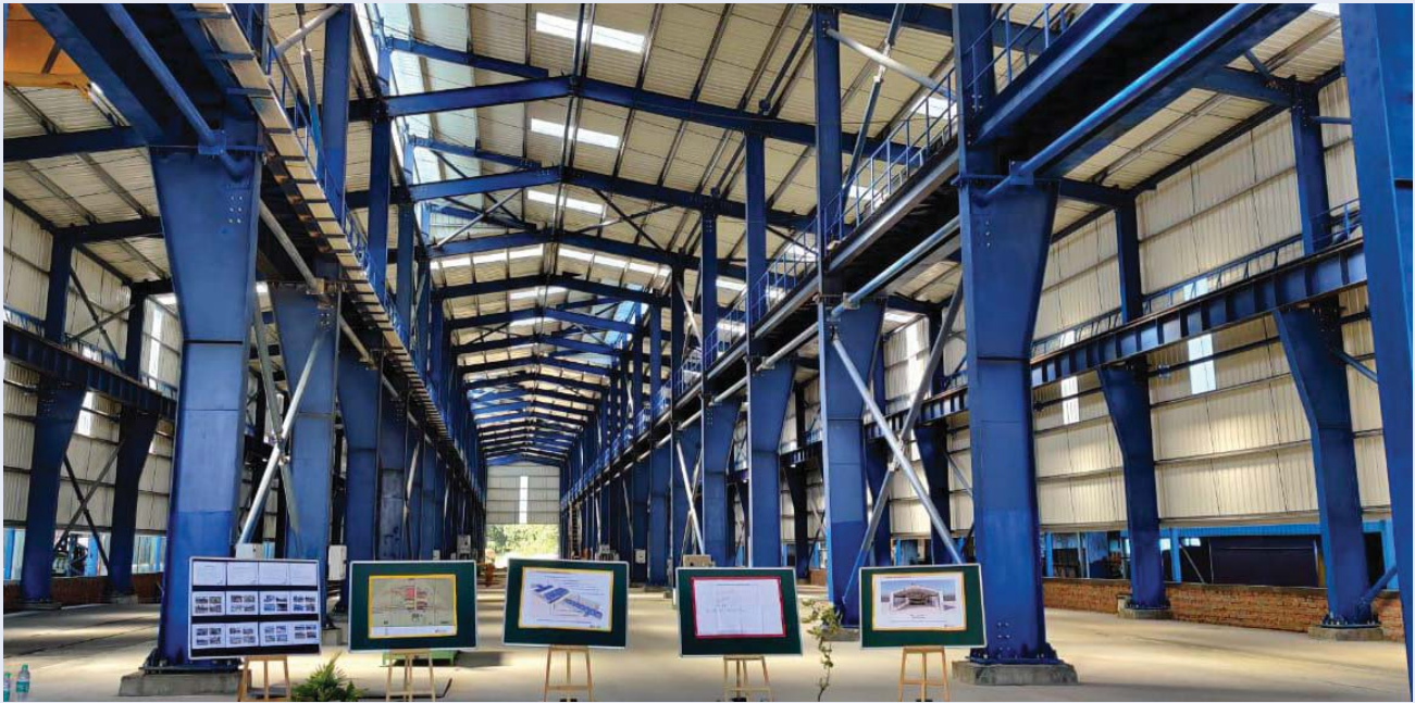
Bogie Repair Shop at New Bongaigaon workshop in Assam
