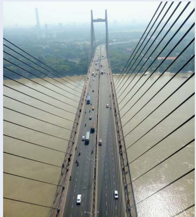
Rehabilitation works for Vidyasagar Setu, India's longest cablestayed bridge
