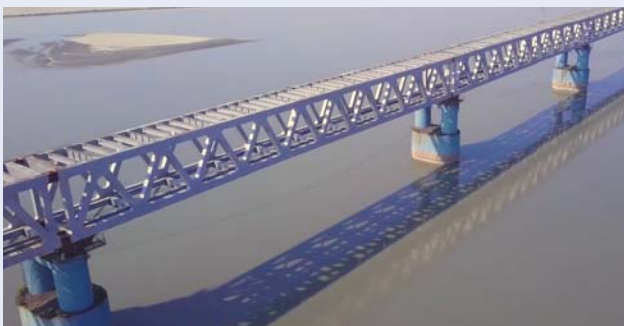
Consultancy for Bogibeel Bridge at Dibrugarh
