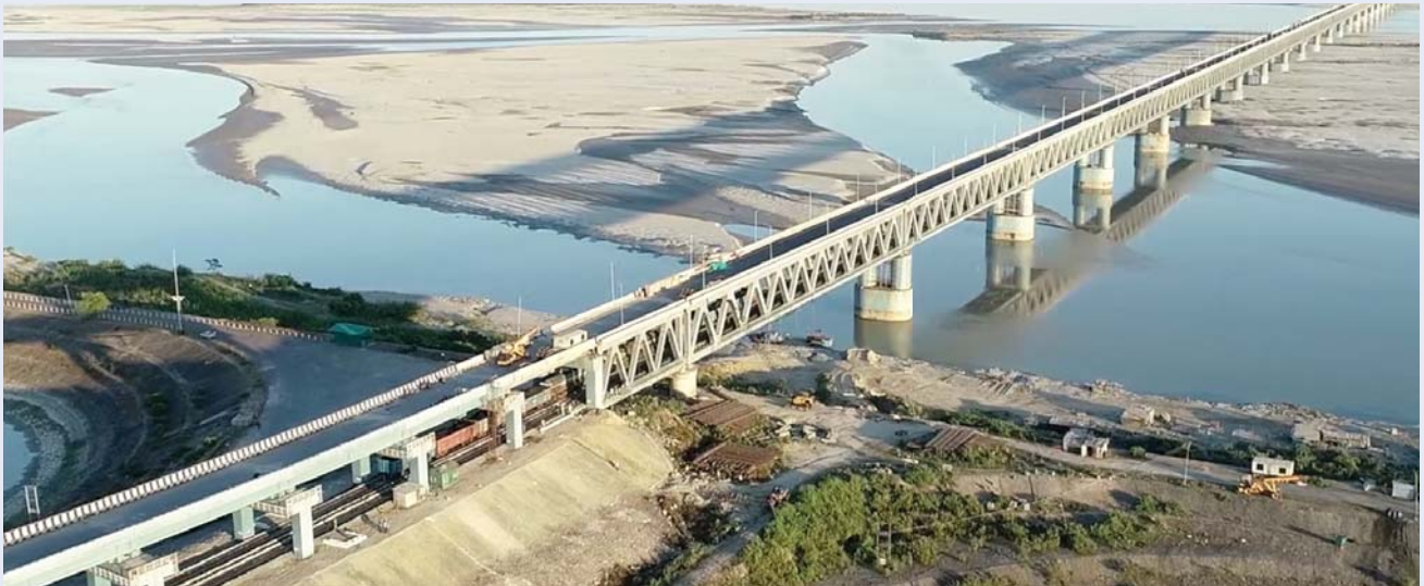
Consultancy services, including structural health monitoring system, for India's longest rail-cum-road bridge, Bogibeel Bridge, over the Brahmaputra at Dibrugarh in Assam
