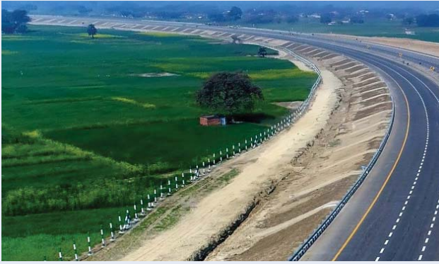
PMC-cum-ETA for Purvanchal Expressway in Uttar Pradesh
